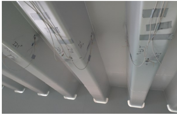
Strain gauges in two cross-sections
