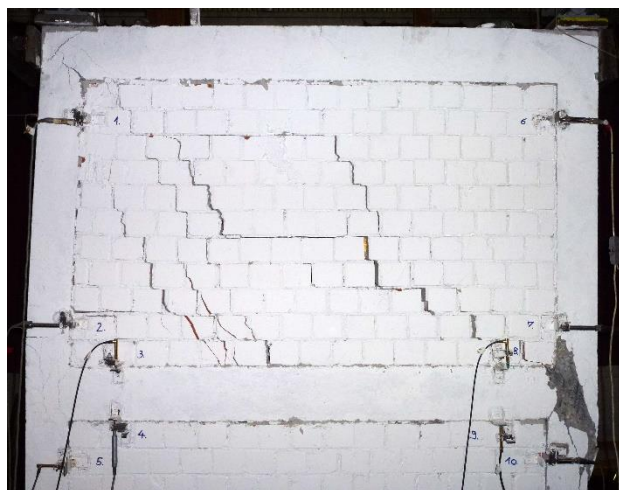
Figure 1.1 Crack pattern of a sheared planar wall in reinforced concrete frame (photo: second author)
